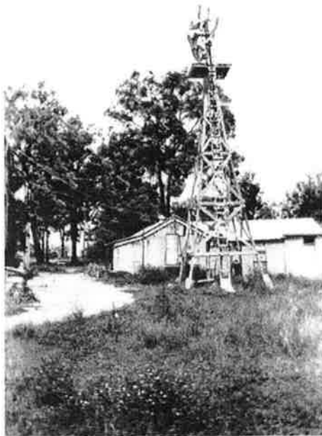
Figure 16 Early windmill and shed on the Grasmere Estate Source: Carrington Archives
