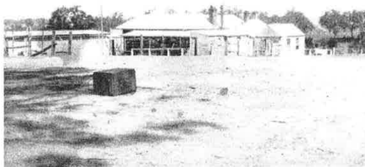
Figure 17 Rear of Grasmere Villa c1930 looking at the northern elevation Source: Carrington Archives
